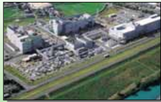
FUJIFILM Opto Materials' facilities in Shizuoka, Japan
