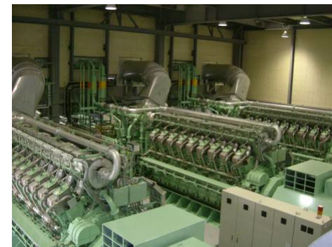
Natural gas cogeneration system (Fujinomiya Factory)
